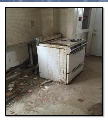
This range is missing parts and is covered with grease which draws bugs and roaches creating a life-safety condition. Removal would be appropriate.
