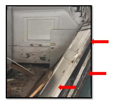
These unattached doors are stacked in a hallway. If doors were in good condition, they would be considered personal property. These have mold on them and should be considered interior debris and a life safety hazard. Vendor can move to garage when in doubt.
