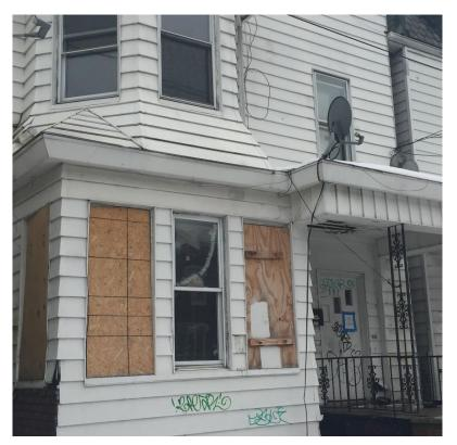
One window boarded with OSB, the other with plywood – both have through bolts and 2 x 4's to secure.
